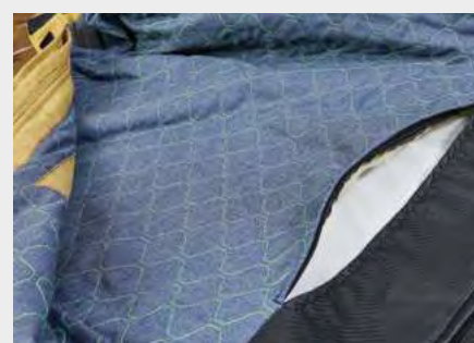
Inspection opening to check the membrane
